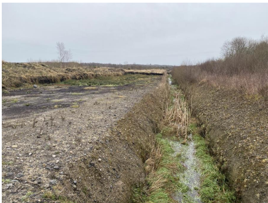
Figure 4 - Exposed glacial till at drain location
